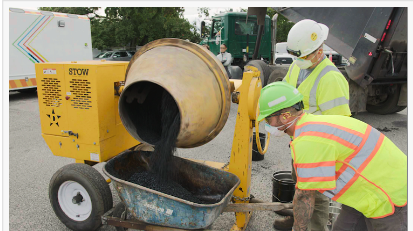
Pavers prepare to use Modern Asphalt in Bellmore, NY, Monday, Sept. 30, 2024
