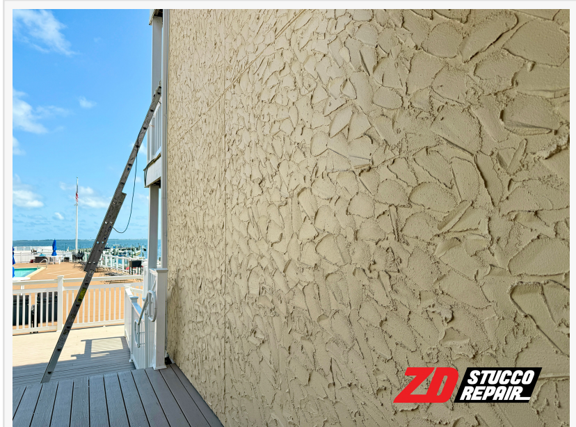
Sophisticated texture restored and matched by ZD Stucco Repair
