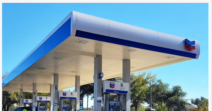
Chevron Fueling Forecourt
