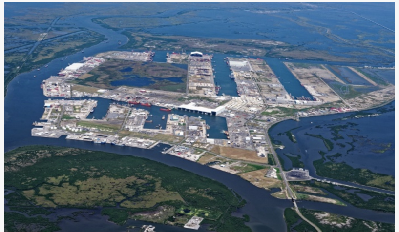
The Greater Lafourche Port
