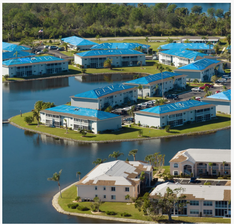
Tarps on roofs after a hurricane
