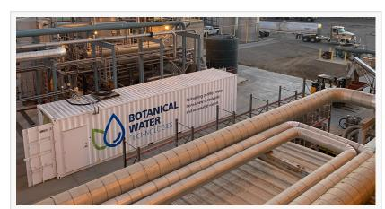
Manufactured, tested, commissioned and serviced, they operate independently to existing equipment. A standard WHU features over 170 "touch points" providing live monitoring and adjustments.
