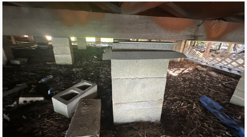
new orleans foundation repair
