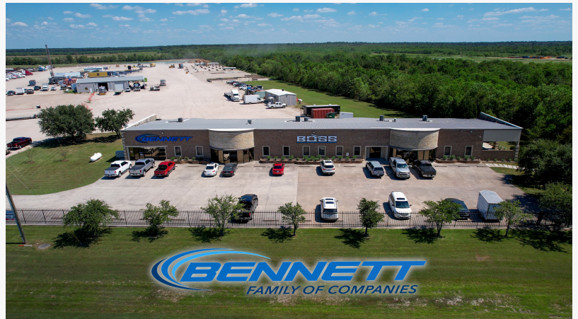
New Dayton, Texas office and yard
