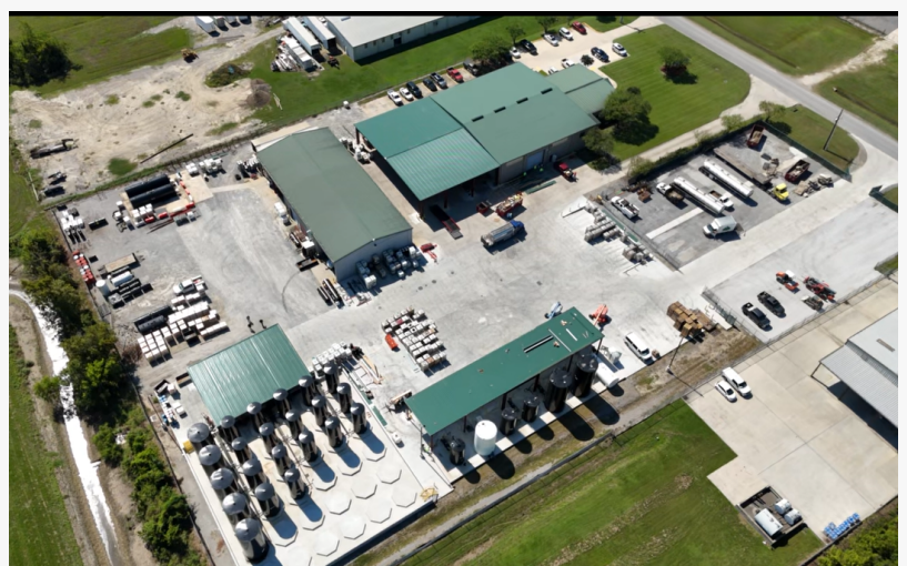
McPherson Bayou Facility
