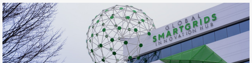
Barbara to Equip Iberdrola with Edge Computing Firmware for Secondary Substations
