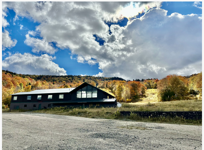
483 Big Tupper Rd, Town of Tupper Lake
