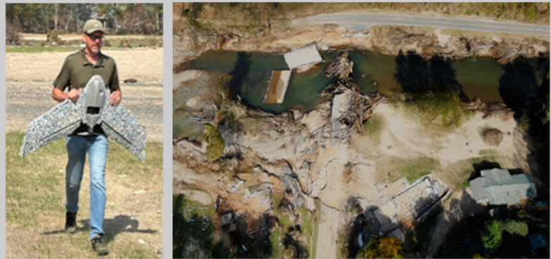
Aaron Schradin shown above with a camera drone that was used to capture footage of bridge that was washed away.
