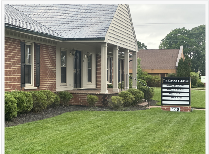
The new office for Randall and Bruch located in Hopewell, VA.
