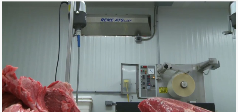
RGF's REME® ATS in Food Processing Plant
