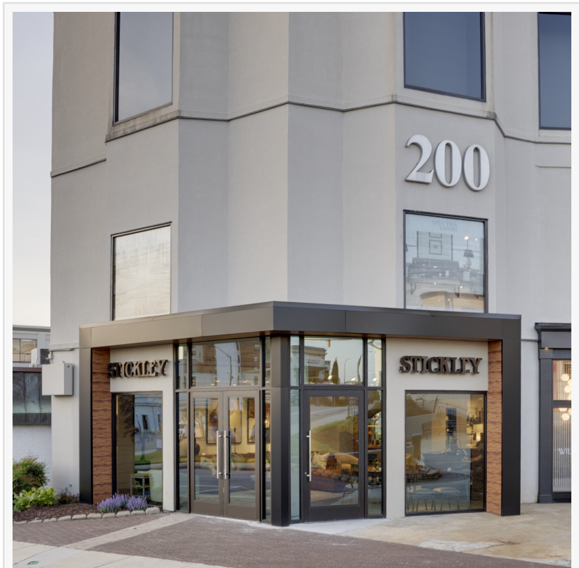
Stickley's home at High Point. 200 North Hamilton Street.
