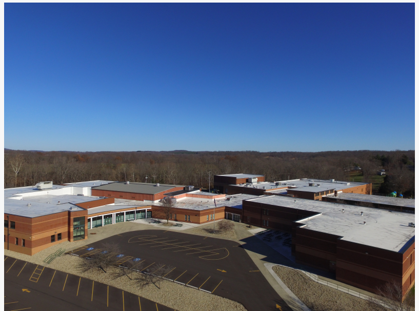
Huntington Local School District located in Chillicothe, Ohio.
