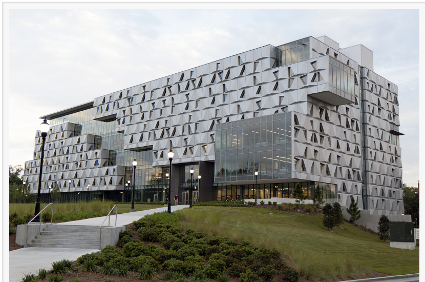
Elevation shot of Malachowsky Hall at the University of Florida demonstrates the ever-changing undulation and play of shadows cast by the volumetric design of the aluminum panels. Photo Credit: N-RG Cladding
