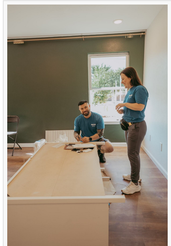
WGU Volunteers Working on Finishing Touches
