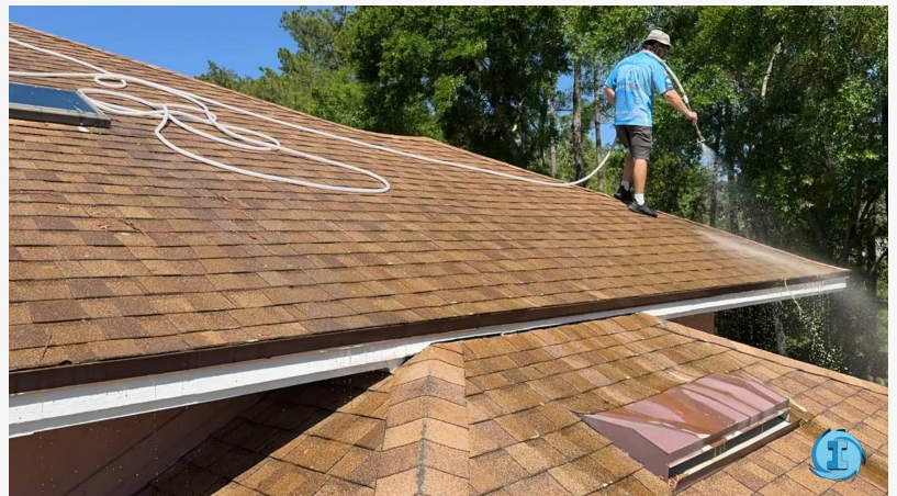
Soft Wash Cleaning a Roof for a Central Florida Homeowner
