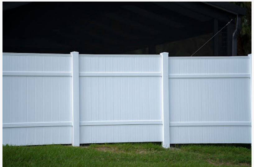
A white vinyl picket fence surrounding a green, well-maintained lawn, providing a secure boundary around the property's backyard area.
