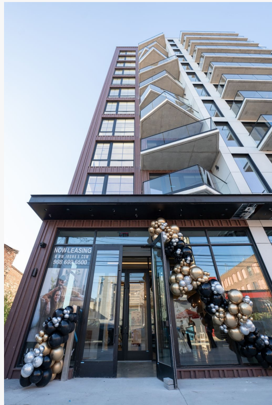
Iron 65: Setting a new standard for luxury living in Newark's Ironbound neighborhood with 135 stunning units.
