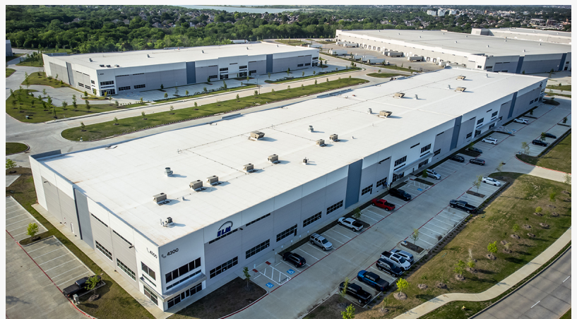
Aerial photo of the ELM MicroGrid
