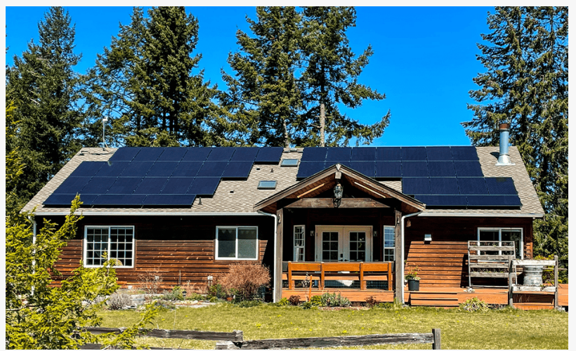
Sunergy Systems Installation
