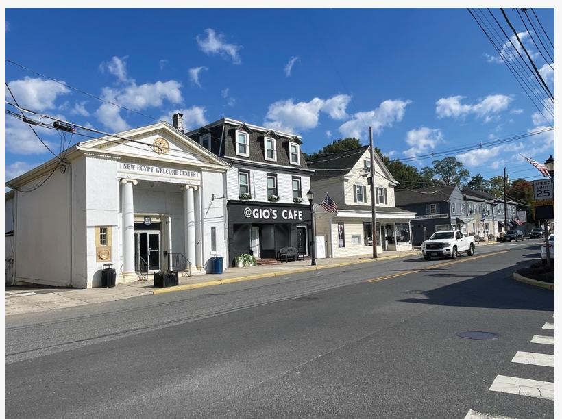
Plumsted Township, NJ Commercial Building on Main Street
