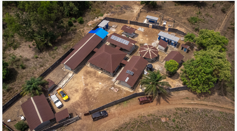
Aerial photo of roof mounted solar panels on Sierra Leonean health facility.
