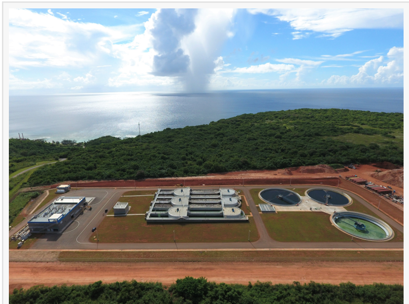
An aerial view of Guam's Northern District Wastewater Treatment Plant, which provides critical wastewater services to two major military bases and the most populous area of Guam.
