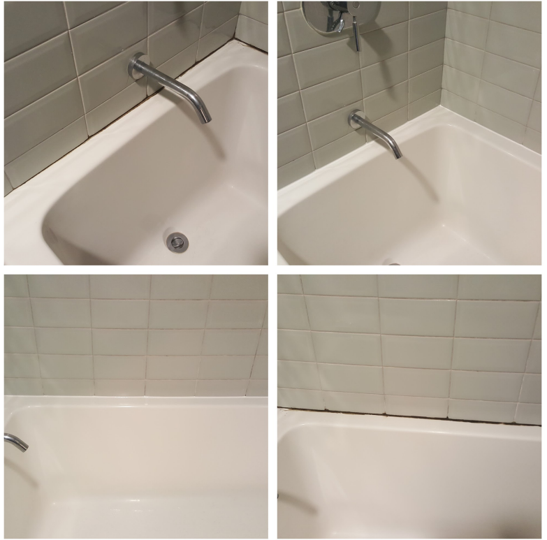
Before and After bathroom shower/tub grouting repair
