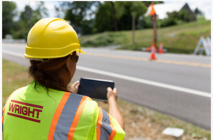
A traffic flagger safely deploys the Guardian SmartFlagger away from traffic using a tablet computer.
