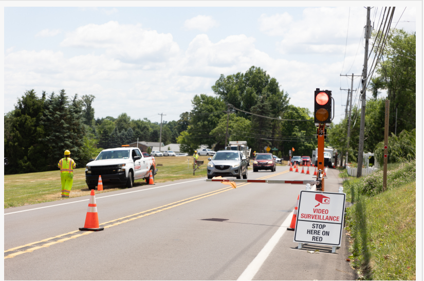
A Guardian SmartFlagger deployed at a road construction site in Pennsylvania.
