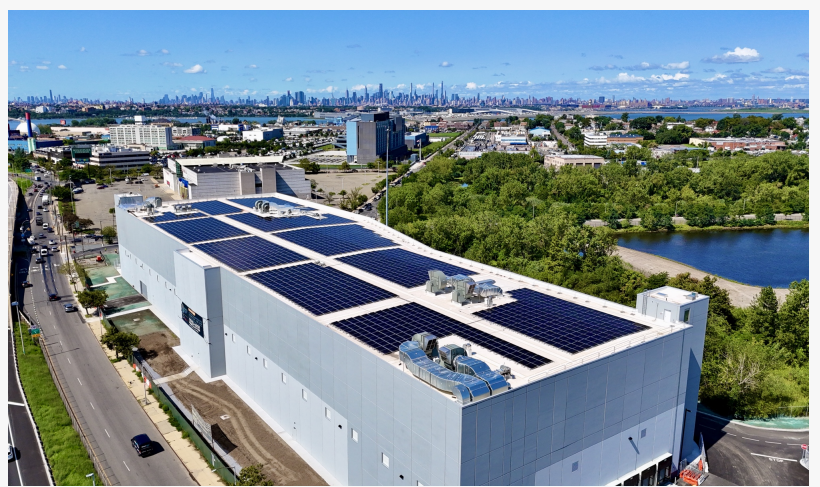
Aerial view of the new Queens project
