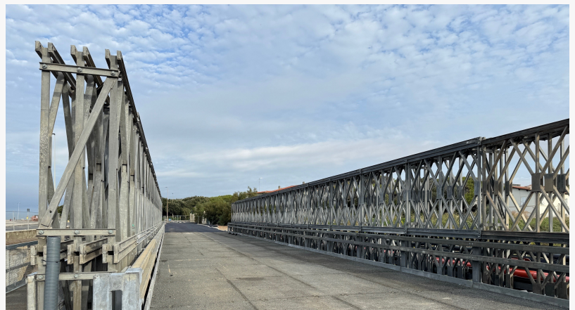
Acrow Bridge in Livorno
