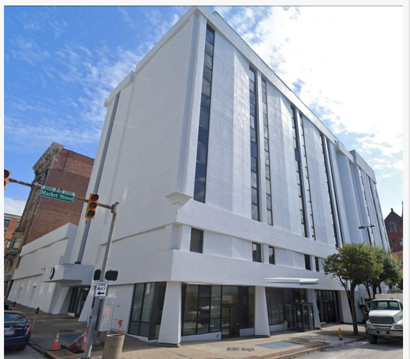
Exterior view of the McLure Hotel
