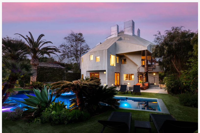
Constellation 167, 167 South Westgate Avenue, Los Angeles, California
