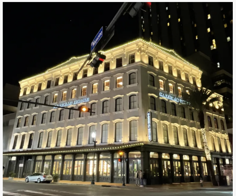
Commercial Christmas Light Installation - Let's Get Lit
