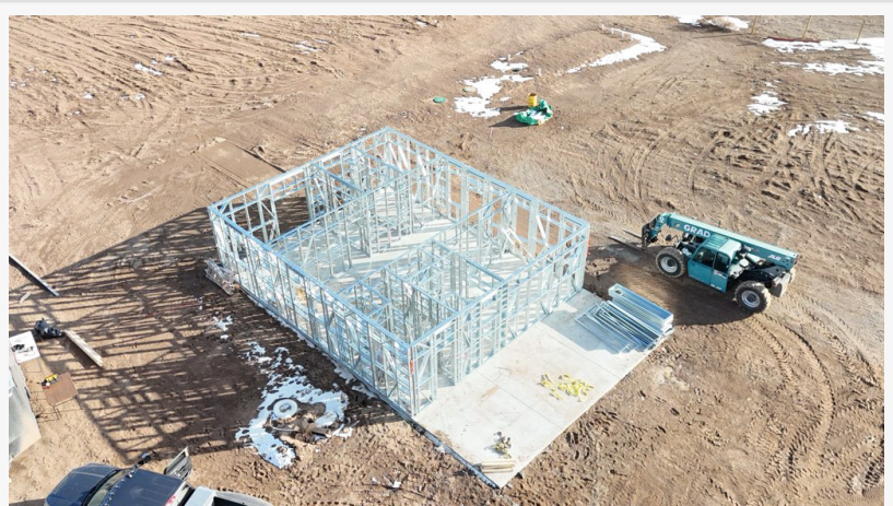
Drone View of Quinn Barndominium being erected
