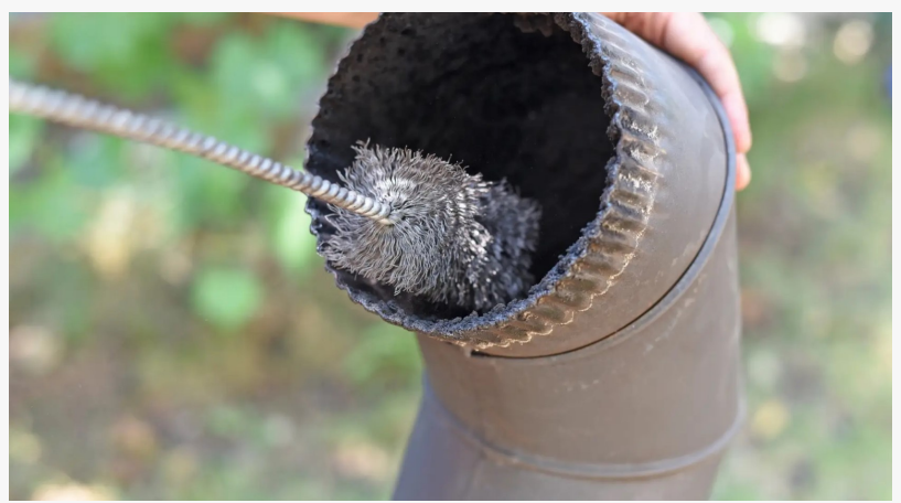
Chimney sweeping in-progress by Fresh Air Duct Cleaning
