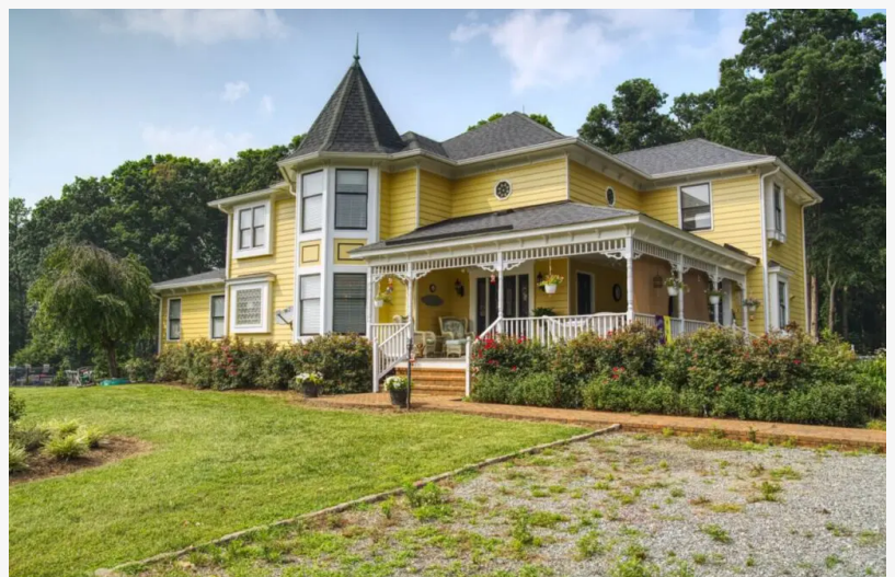
Exterior Painting Richmond
