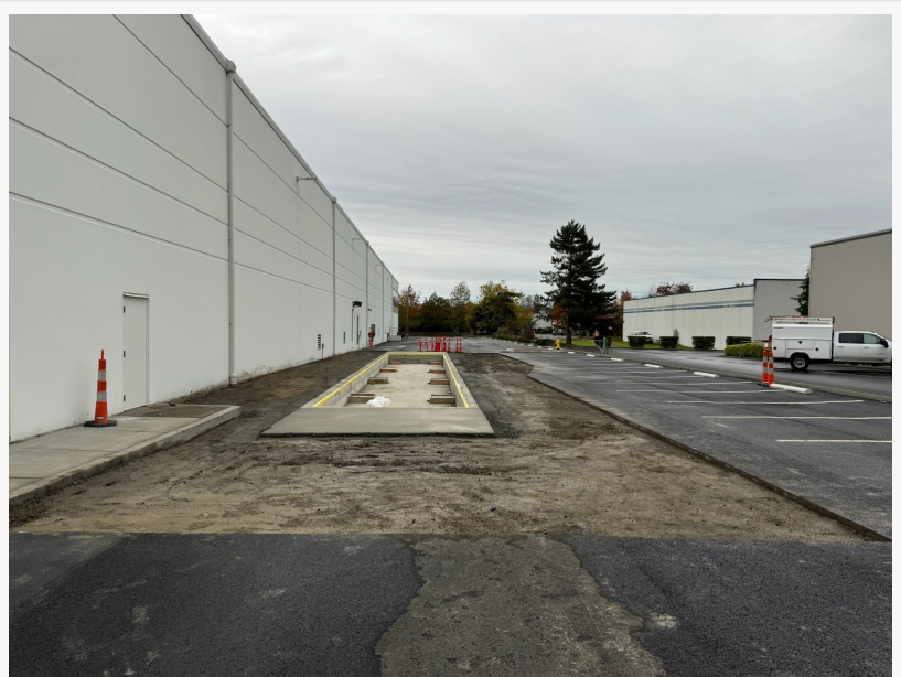
Weight Scale for Trucks Excavation Project in Tacoma, WA
