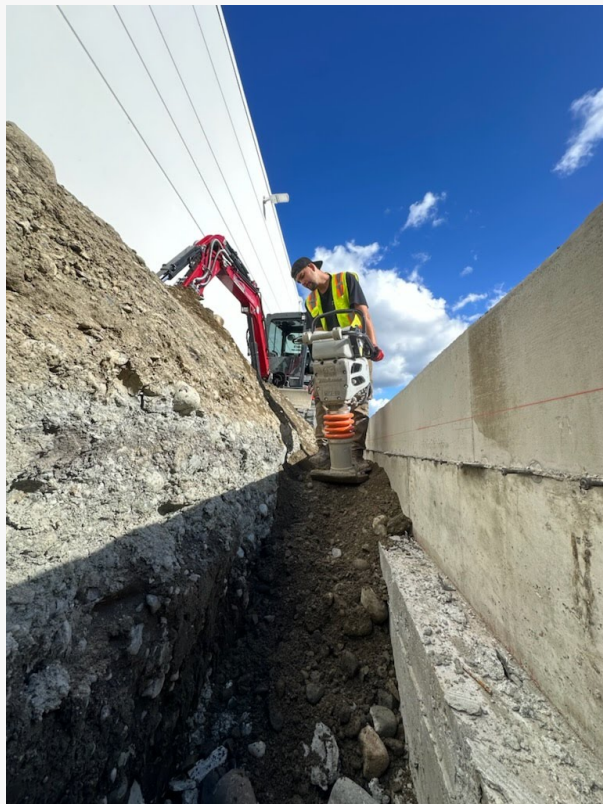
Excavation for Utilities Job in Tacoma Washington
