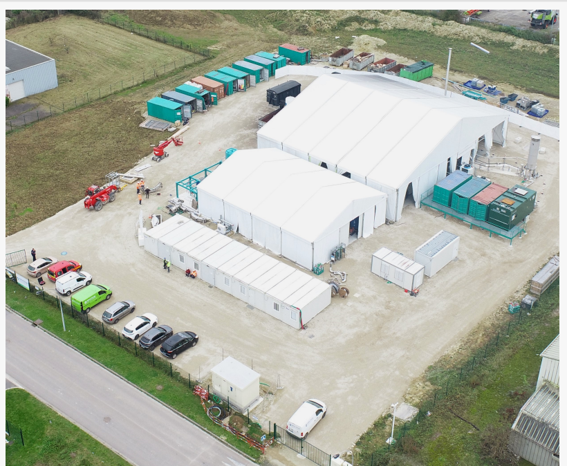
Haffner Energy's center of hydrogen production, testing and training in Vitry-Marolles industrial zone, Marne County.
