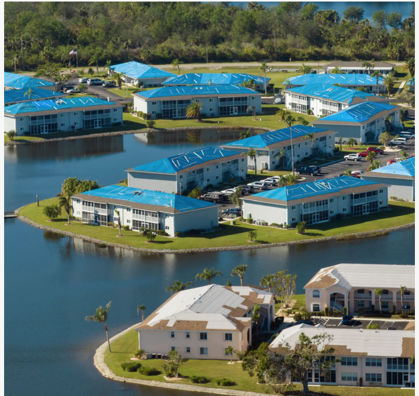
Tarps on roofs after a hurricane
