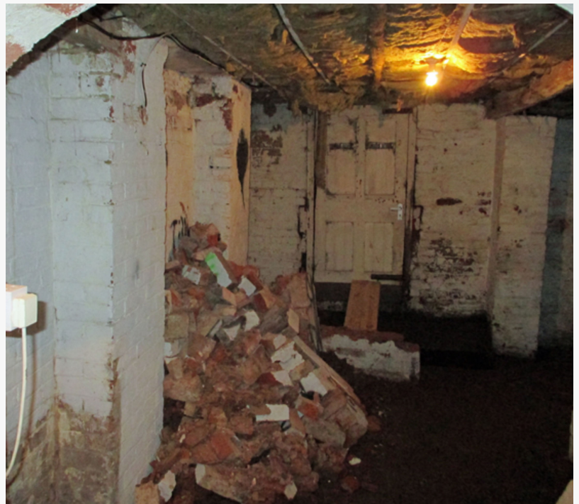
Cellar Conversion Waterproofing
