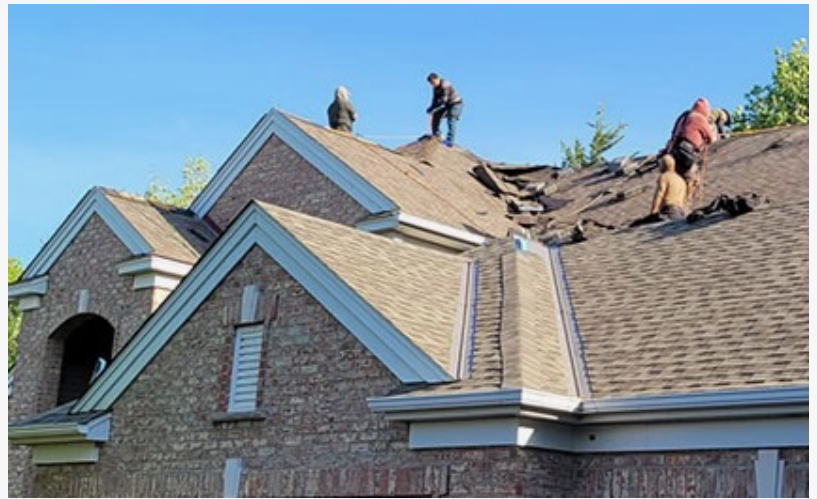
Wolf River Construction Reroof
