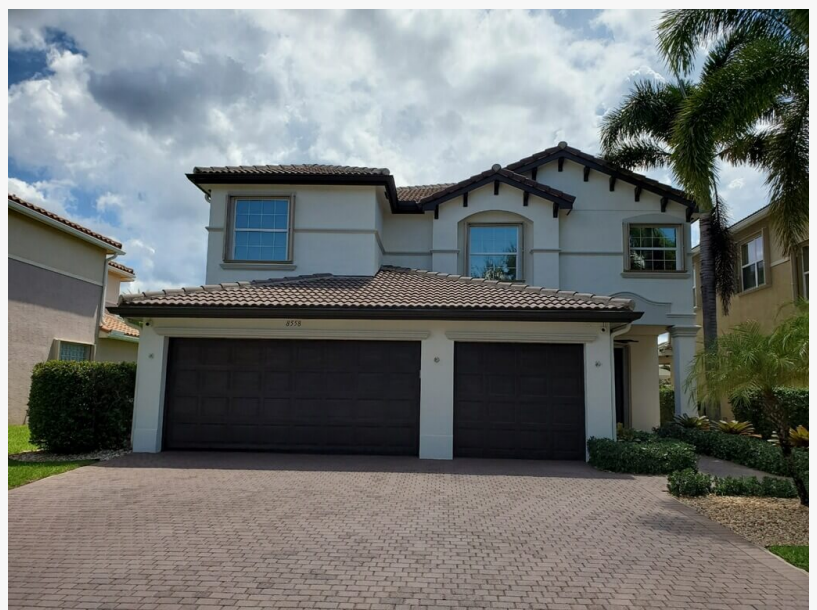
Boynton Exterior Painting
