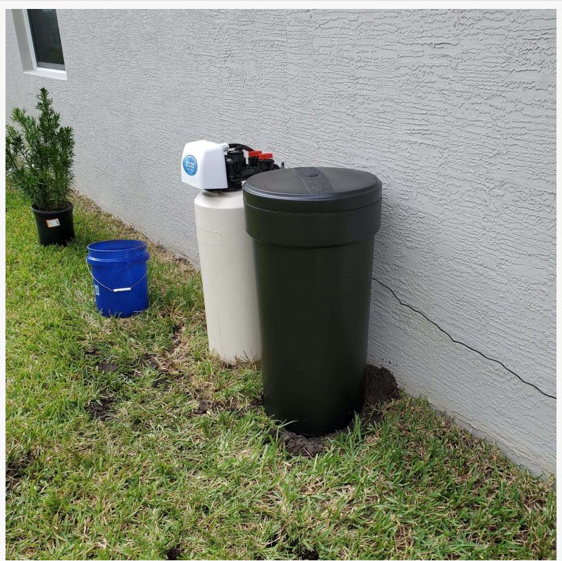
PSL Water Guy's carbon filter removing chlorine in Port St. Lucie.
