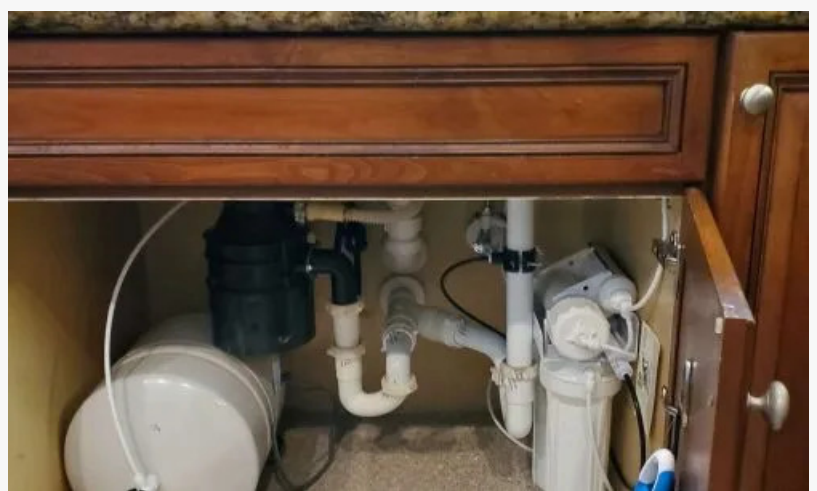
PSL Water Guy installing advanced reverse osmosis filter.
