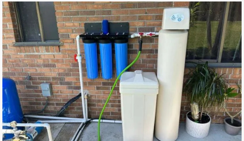
Technician installing water filter for clean water.
