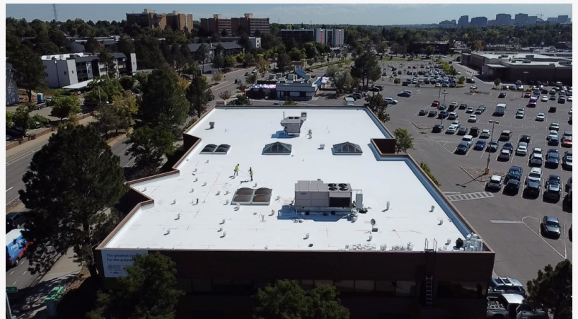
Roof Coating Project
