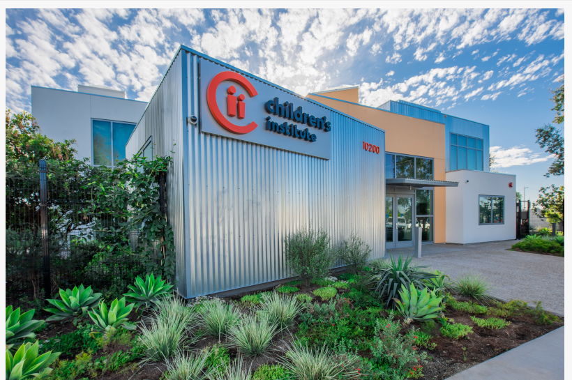
Children's Institute's campus in Watts, designed by the legendary architect, Frank Gehry.
