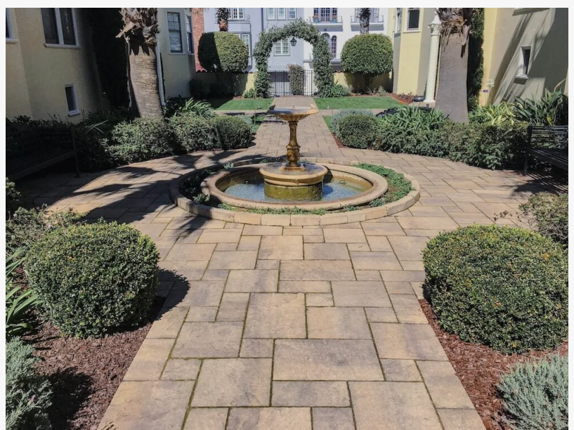
Paver Installation Napa
