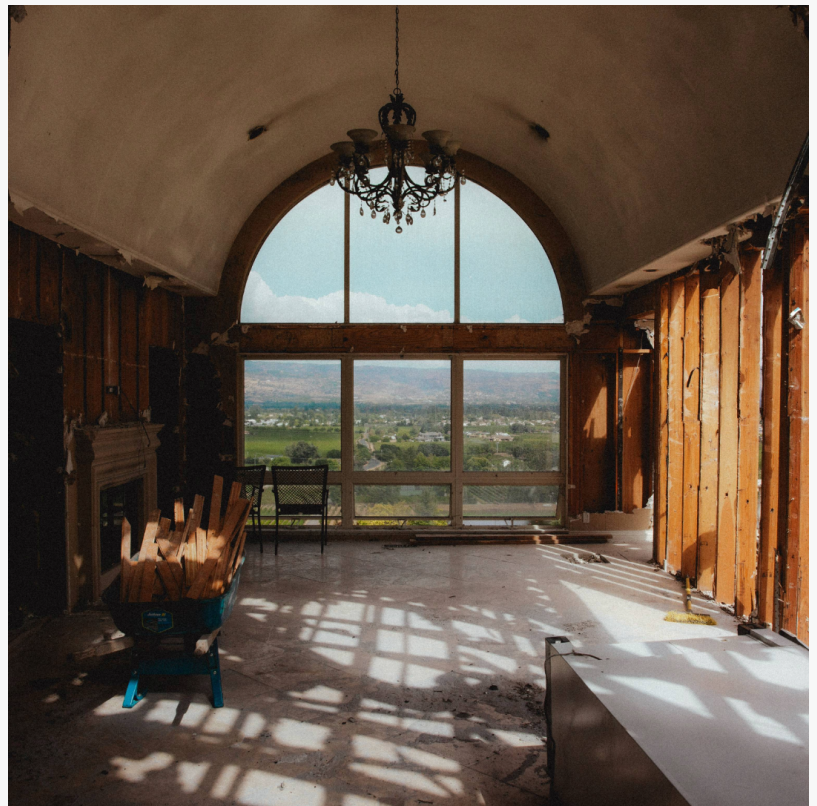
Interior Demolition Sonoma
