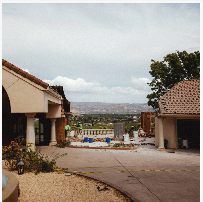
Exterior Demolition Sonoma
