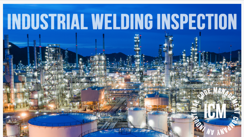
Industrial Welding Inspection Service in Southwestern United States
