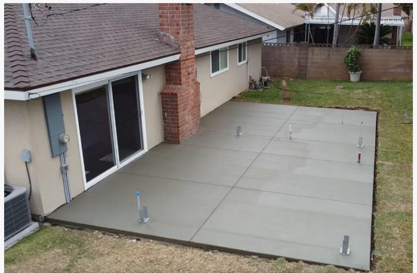
Concrete Contractor Company Columbia, MD
