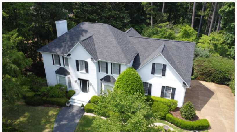
A premium roof replacement
