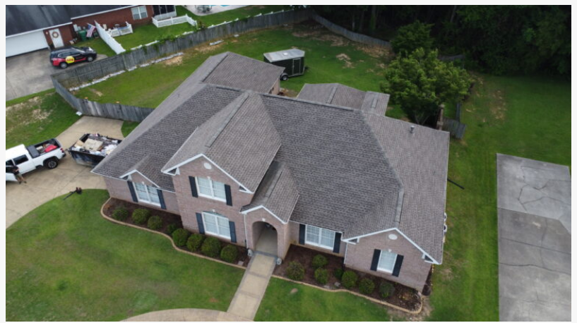
An overhead drone picture of a finished roof in Birmingham, AL
